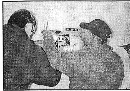
Mike Ray and Ian Hill installing interp. panel in plotting room.
